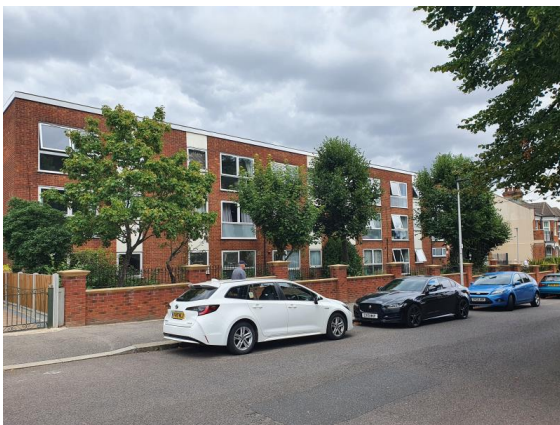
Front view 1-20 Highland
