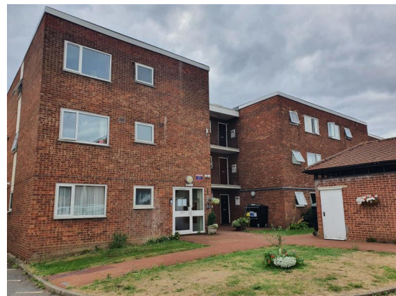
Rear view 1-20 Highland
